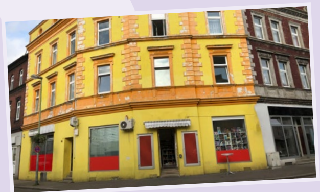
Problemimmobilie in Essen
