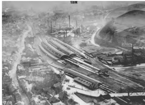
1926 Aerial view of the station district
